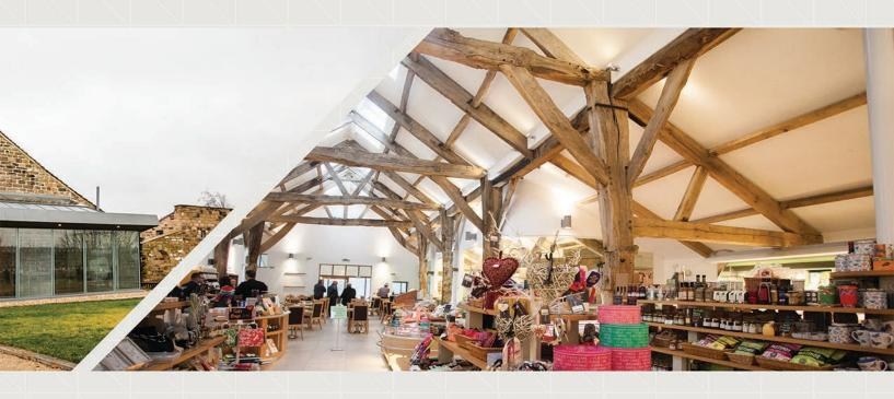
The tin roof was stripped from the building, the roof structure replaced and a traditional Yorkshire stone roof reintroduced. Under floor heating was added and the walls insulated using sheep's wool insulation, wood wool boards and finished the traditional lime readers. To complement the historic structure we added two contemporary structural glass extensions
